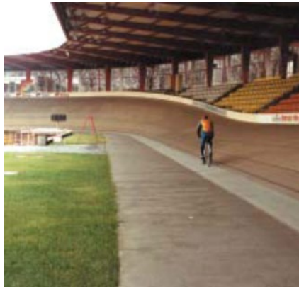
Figure 4: Semi covered track in Germany
